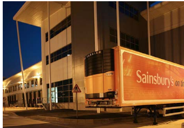
Prologis Park Pineham, Northampton, United Kingdom
